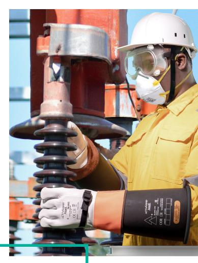
In the case of hand protection, opt for industrial rubber insulating gloves (RIGs) designed specifically for electrical hazards.
